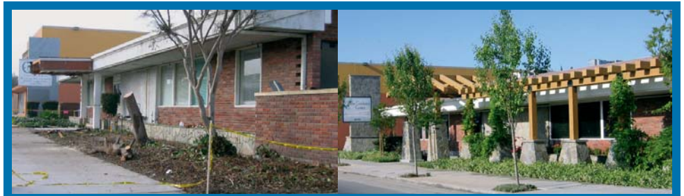
ADMINISTRATION OFFICE BEFORE AND AFTER
